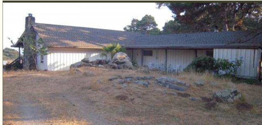
The Science Room & King Room
